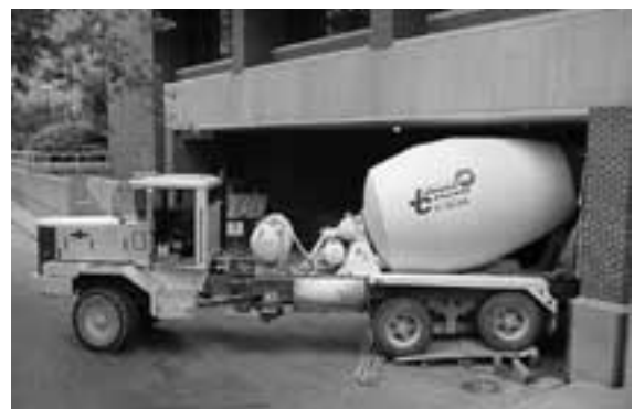
One of dozens of cement trucks involved in the basement buildout project.
